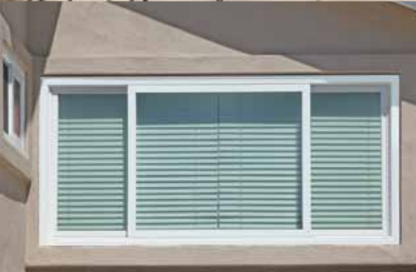
Double slider with Z-bar on stucco
